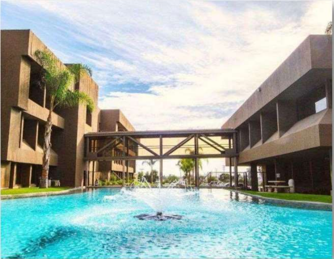
AUHS Building 2 and 3
